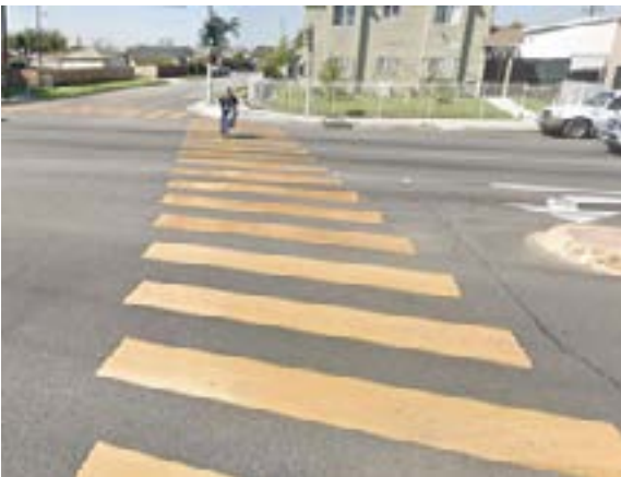
An example of a high-visibility continental crosswalk
