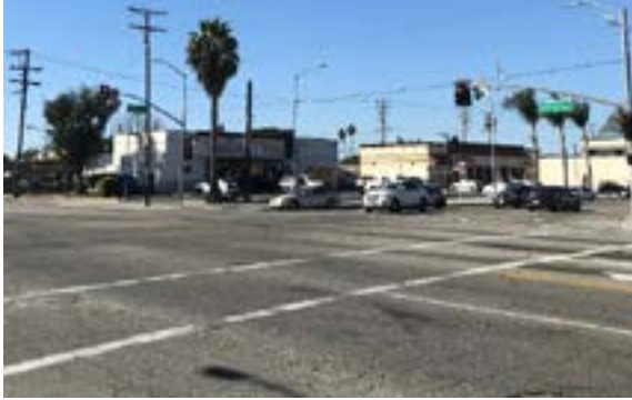
A standard crosswalk with parallel lines on Atlantic Avenue
