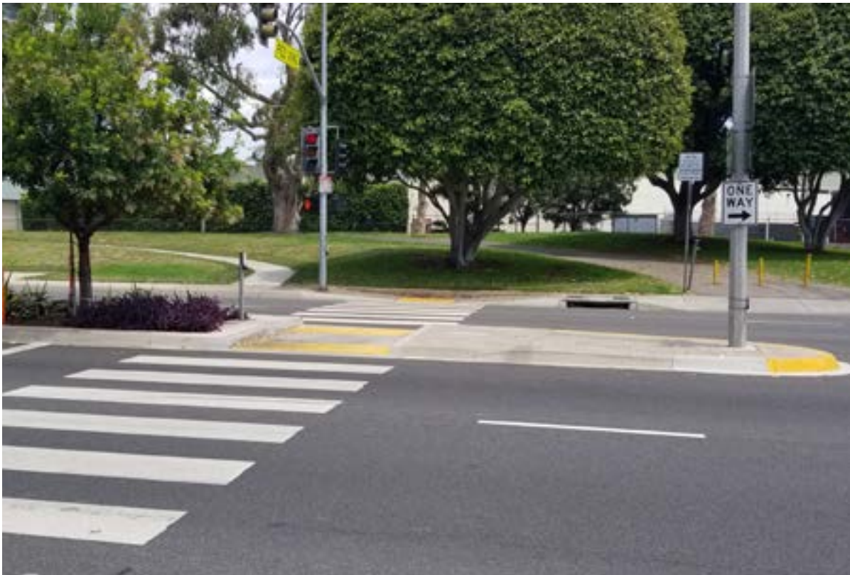
A median refuge island at a marked crosswalk with pedestrian crossing signage
