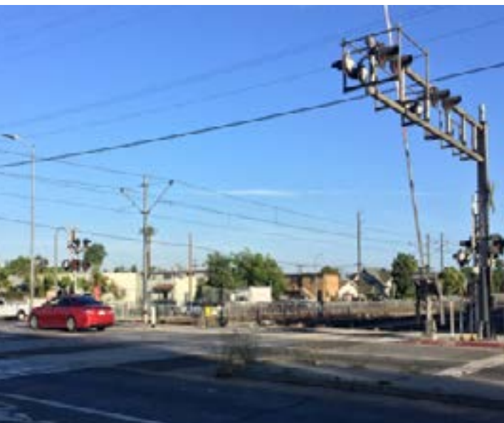
Intersection of 92nd Street and Graham Avenue. Photo Submitted by Yanel Saenz, CAC Member and Florence-Firestone Resident
