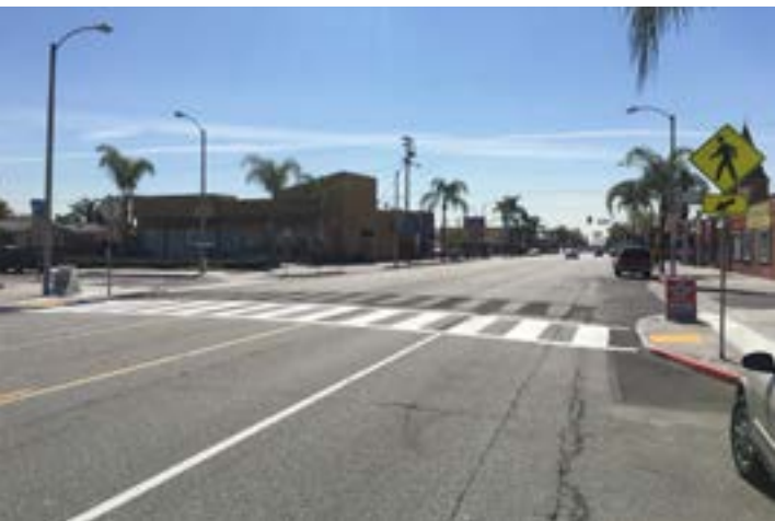
A ladder crosswalk with accessible curb ramps and curb extensions in Walnut Park
